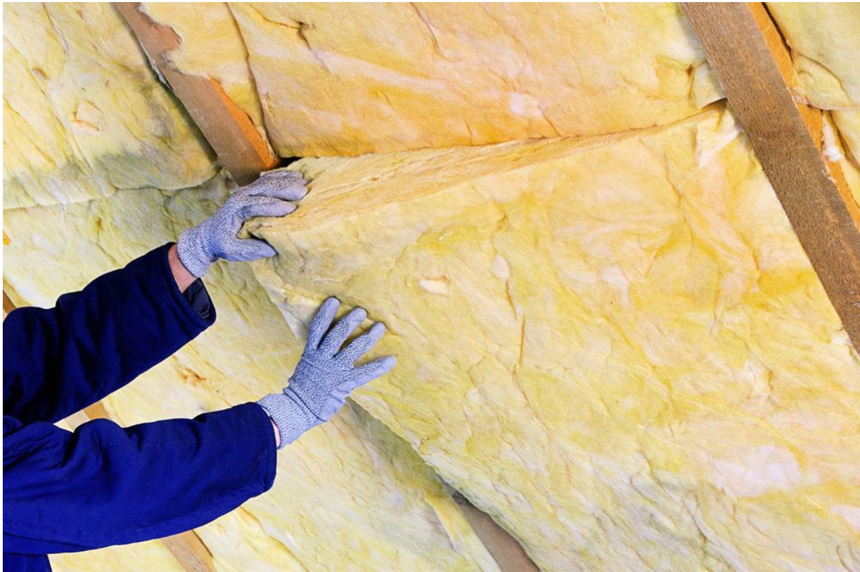
Figure 3: Safety Precautions with Stone Wool Installation
